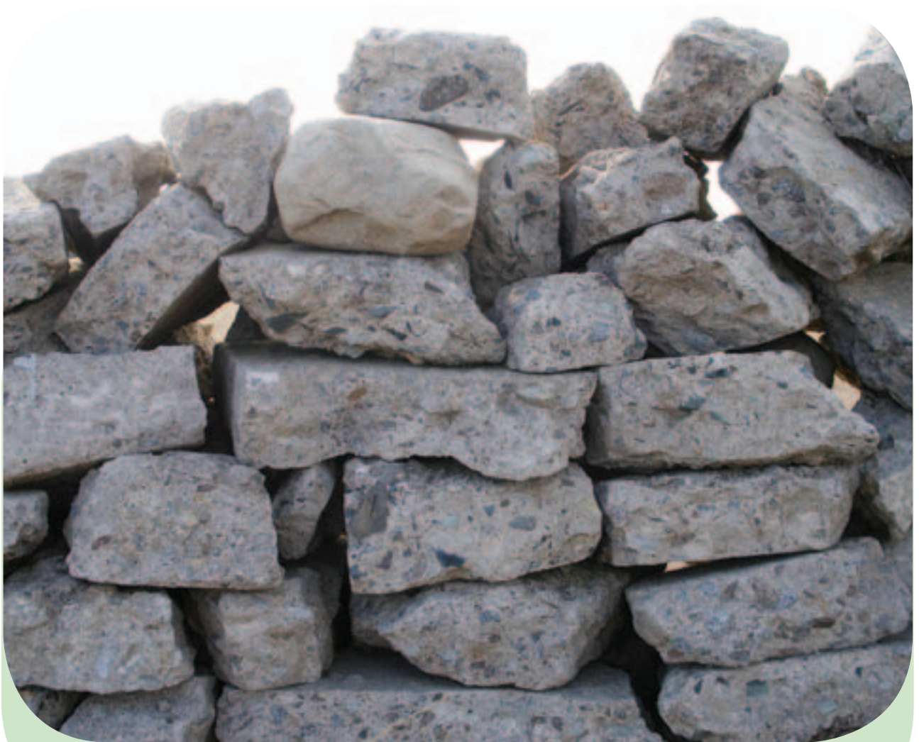
Figure 59 Dry ‘stone’ wall made of broken concrete slabs lifted from a local WW2 airfield.
